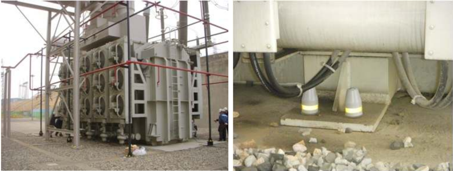
Reinforcement of the Anchorages of Main Transformers
